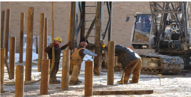
Piles are driven in the area of the future auditorium
