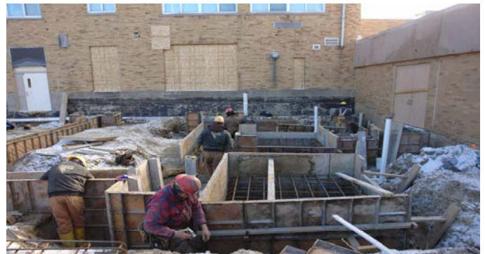
Workers set the forms prior to pouring the foundation
